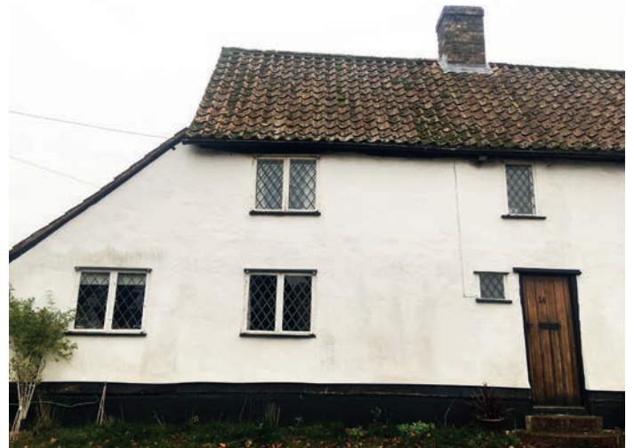
Fig 15 Rendered Church End cottage with black pitch plinth and catslide pantile roof
