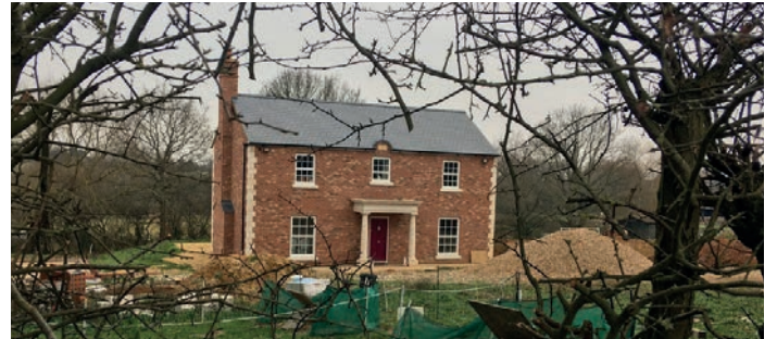
Fig 27 New house nearing completion, Little Heath
