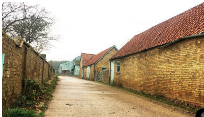
Fig 45 View through Church End long plot
