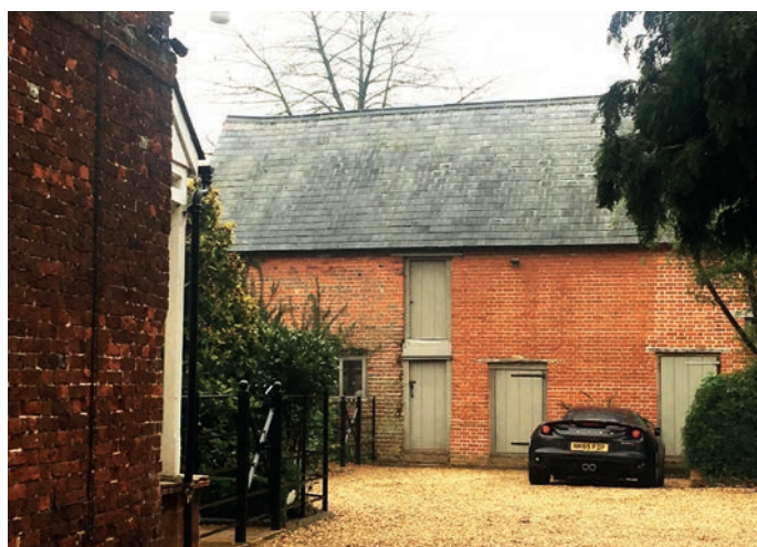
Fig 55 Brick and slate agricultural building
