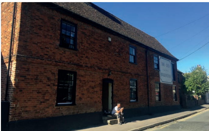
Fig 41 The Old Bakery, Mill Street, sits tight to the pavement just before the Church Street junction
