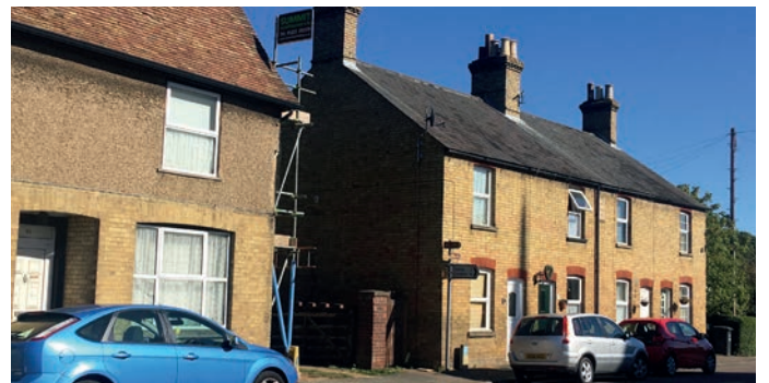
Fig 21 Terraces tight to back of pavement line
