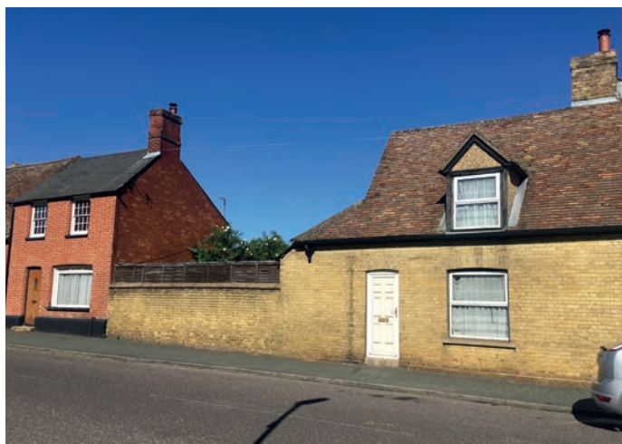
Fig 54 Church Street, Variation in form of clay and slate roofs including dormers and hips.
