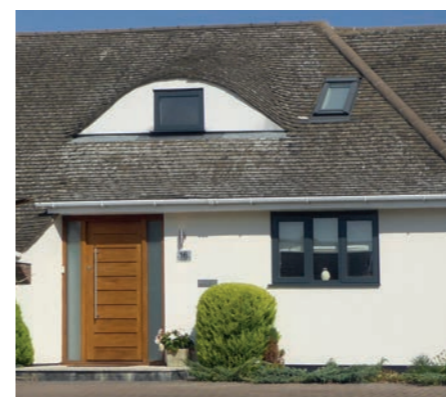
Fig. 36 - Upgraded doors and windows in contemporary style
