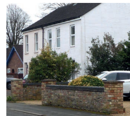
Fig. 37 - Car parking concealed behind walls and hedges
