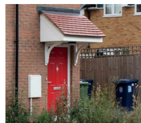
Fig. 73 - Prominent electric box and heavy porch detail can spoil a facade
