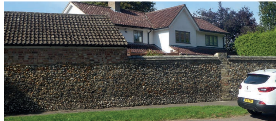
Fig. 54 - Traditional brick and flint walls - a distinctive feature of the village - used to define the edge of private spaces
