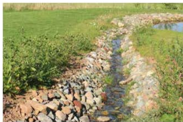
Fig.21 Example of an attractive rural SUDS system within a larger new development. The typical Caldecote ditch is deeper than this example and its banks are greener.
