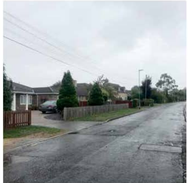
Fig. 12 A typical Highfields streetscape.
