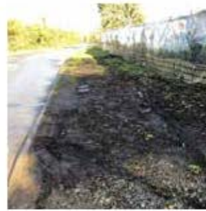
Fig. 9 Highfields Road: 'There is no pathway here, where new housing is coming. Pedestrians have nowhere to go, which is particularly bad for buggies.'
