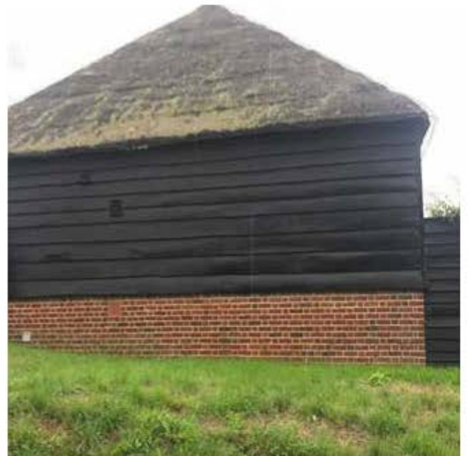
A more 'rustic' approach to timber cladding used in Caldecote village. This resonates with the village's agricultural character.
