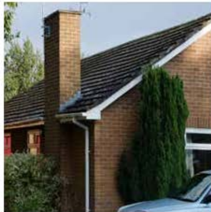
Brick tends to be treated simply, without complicated detailing or patterns. Bricks in white, yellow, buff and red are used throughout.
