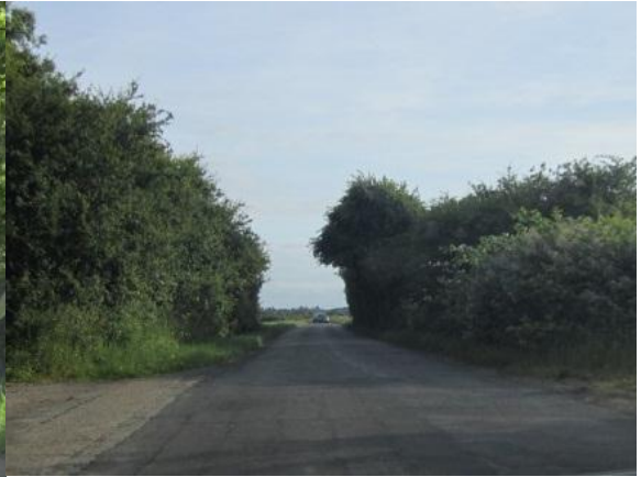
Photo 3.7 – Longstanton Road (Airfield Road)
