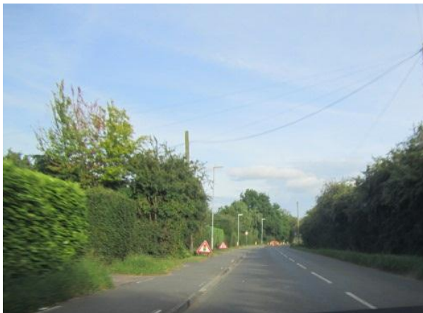
Photo 2.13 – Footway / Cycleway – northern side of Cambridge Road (Cycle Route 24)
