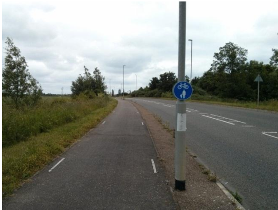
Photo 2.11 – Footway / Cycleway – Hatton’s Road
