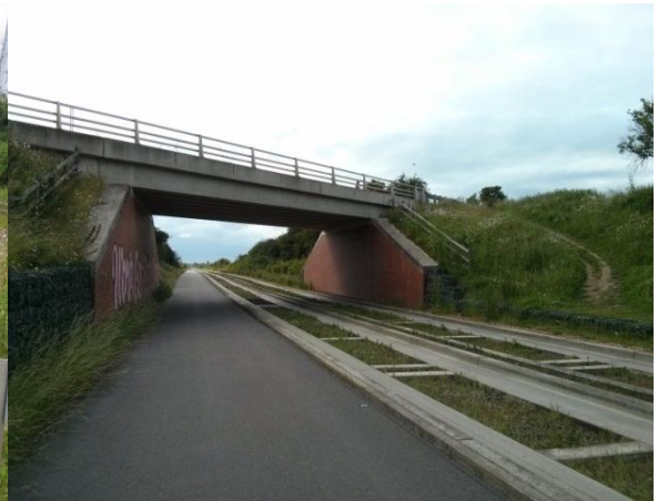
Photo 2.8 - Access to busway from Over over bridge
