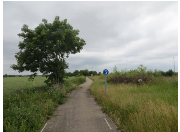
Photo 2.12 - Footway / Cycleway – Hatton’s Road
