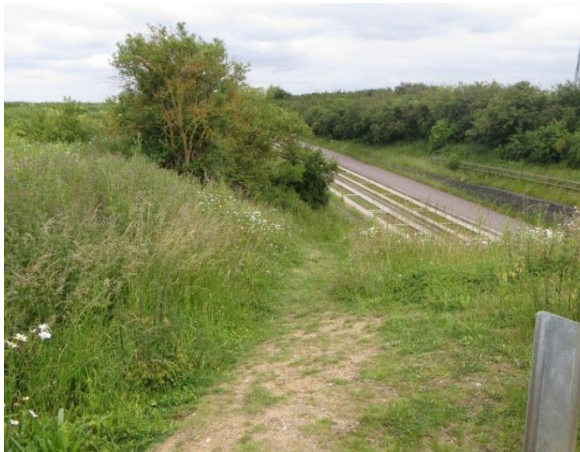
Photo 2.7 – Access to busway from Over over bridge
