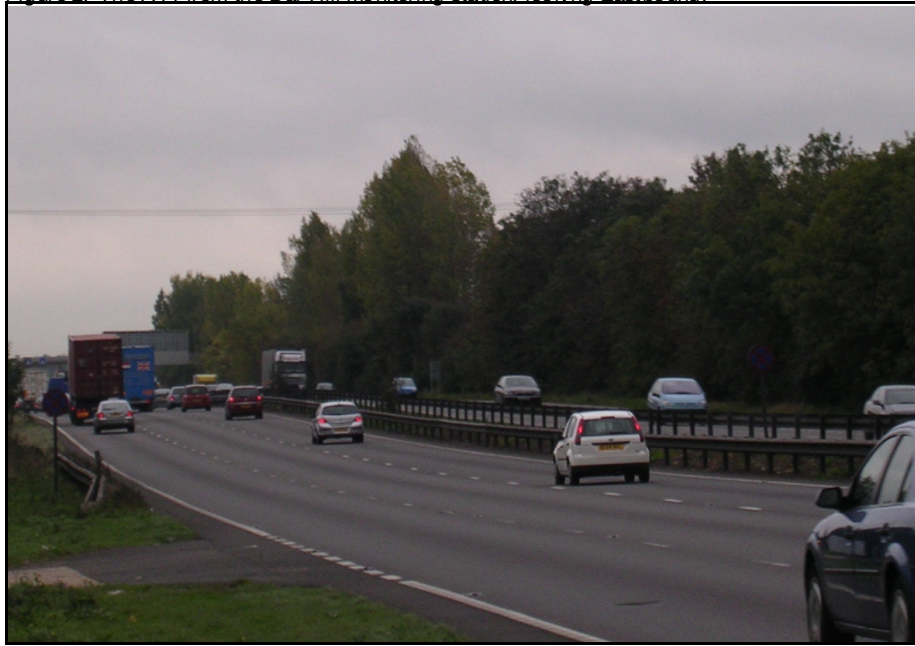
Figure 2: The A14 from the Bar Hill monitoring station, looking Eastbound.
